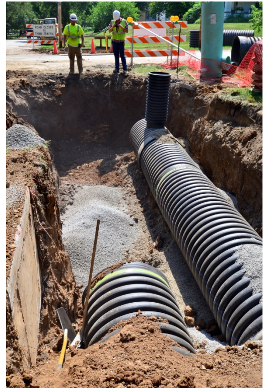
Figure 14 Subsurface Storage Vault
