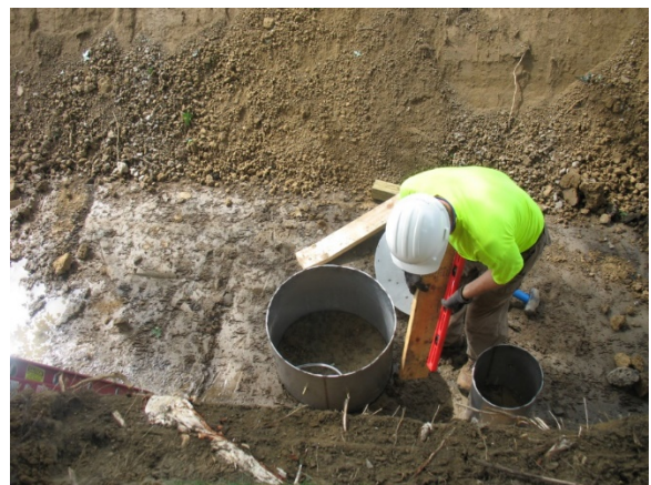
Figure 16 Subgrade Infiltration Test
