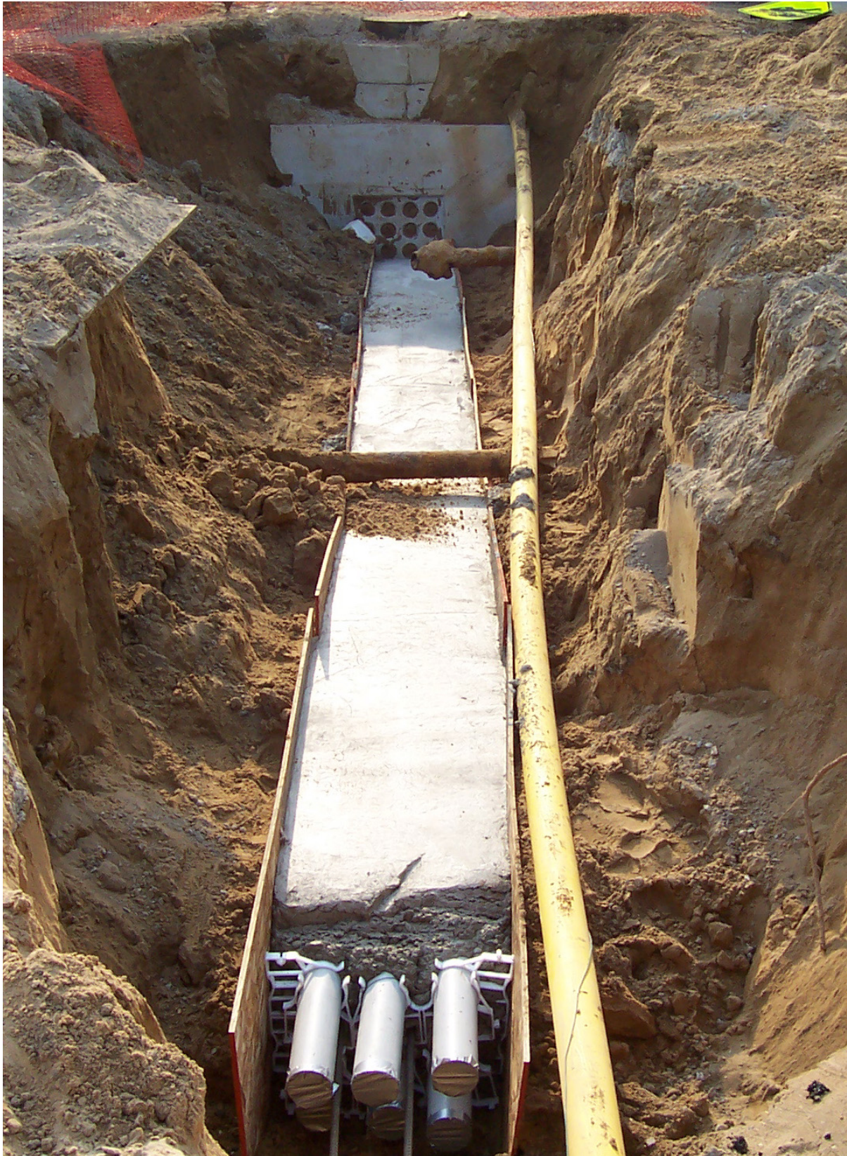
P6 Duct Installation in Wealthy Street
