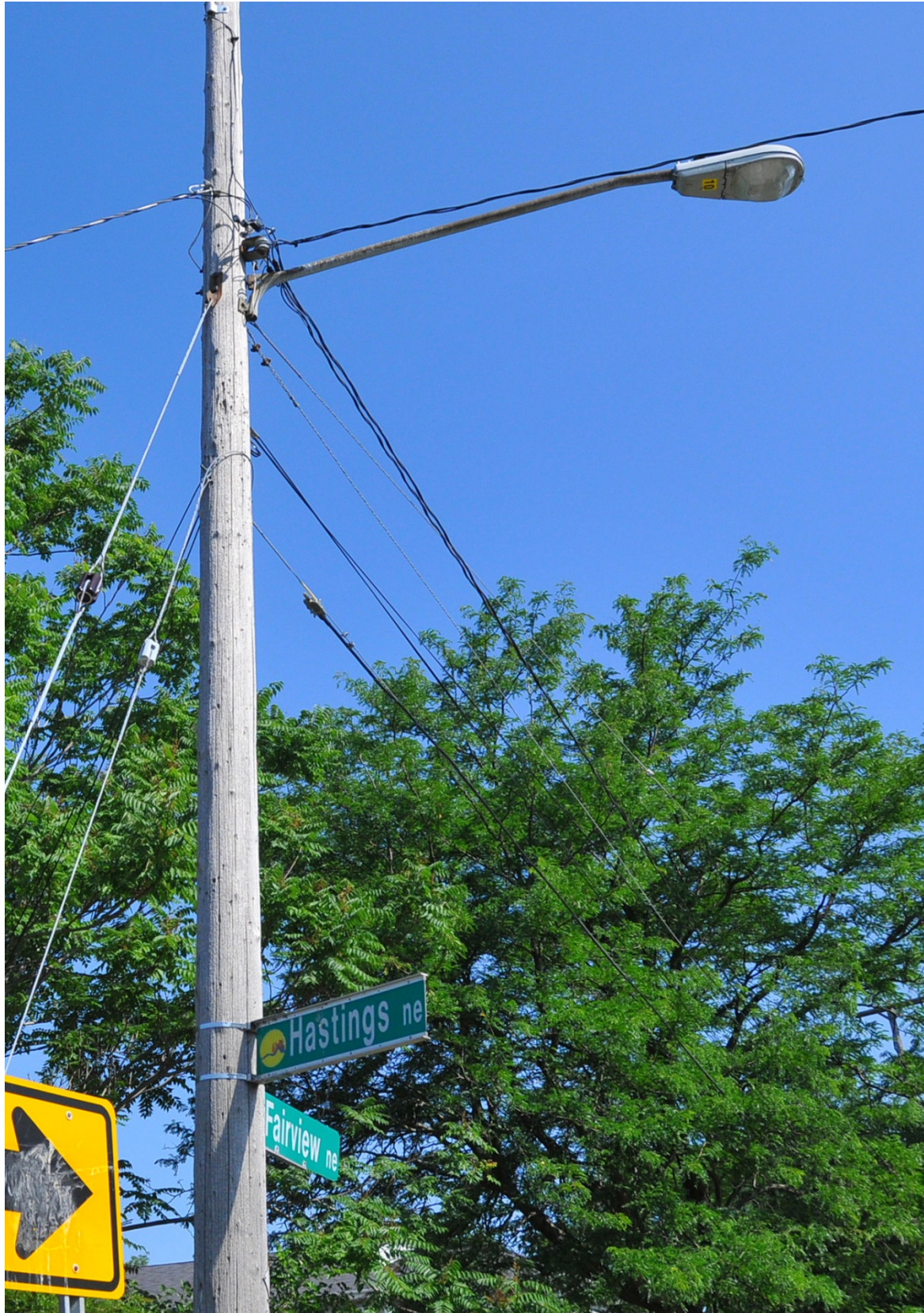
P1 Wood Pole with Cobra Head Luminaire
