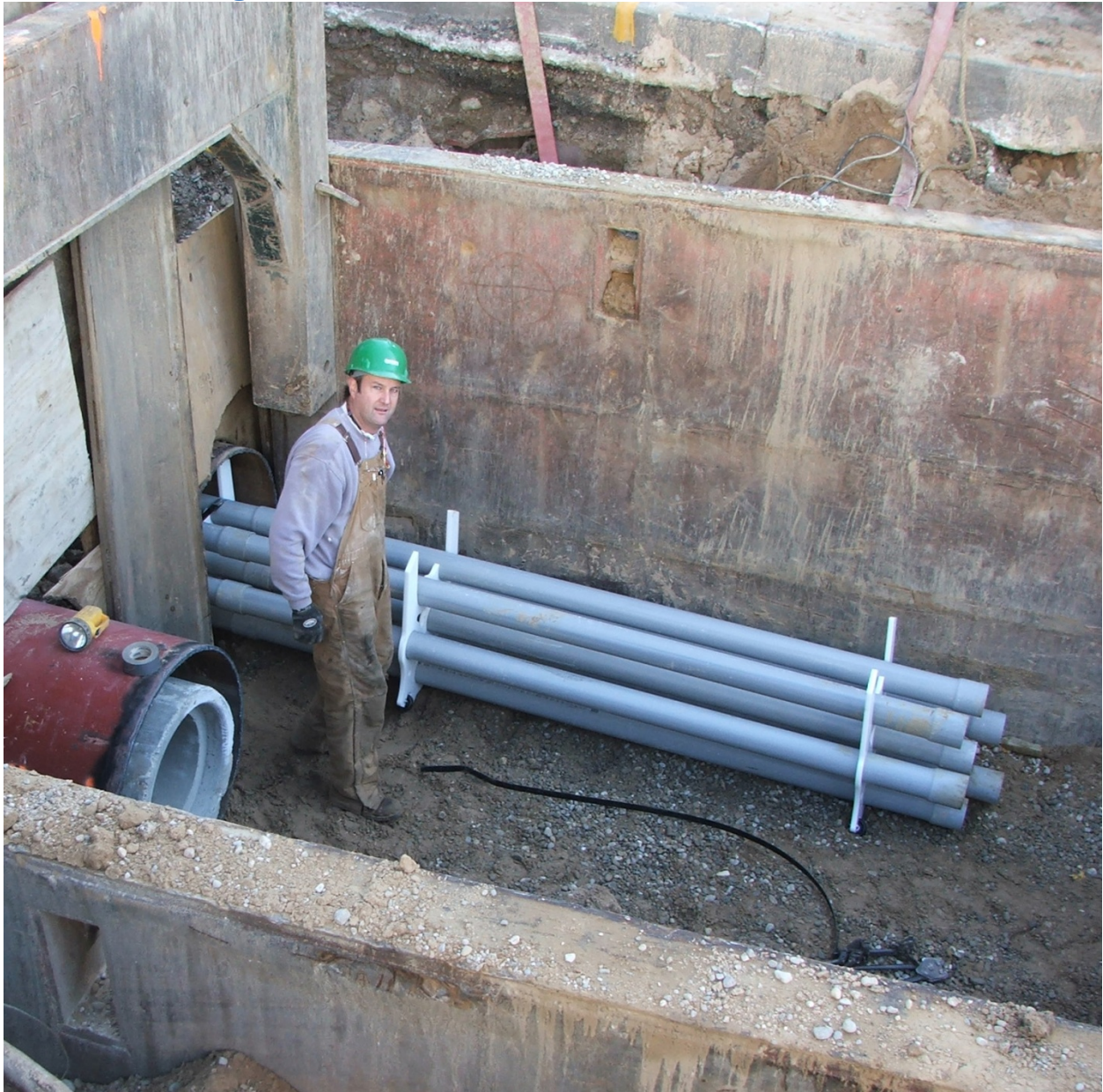
P5 Duct alongside Storm Sewer under US131
