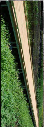
PROPOSED PILE-SUPPORTED BOARDWALK WITH RECYCLED PLASTIC DECKING AND BUMPER RAIL - 12"-.18" ABOVE GRADE
