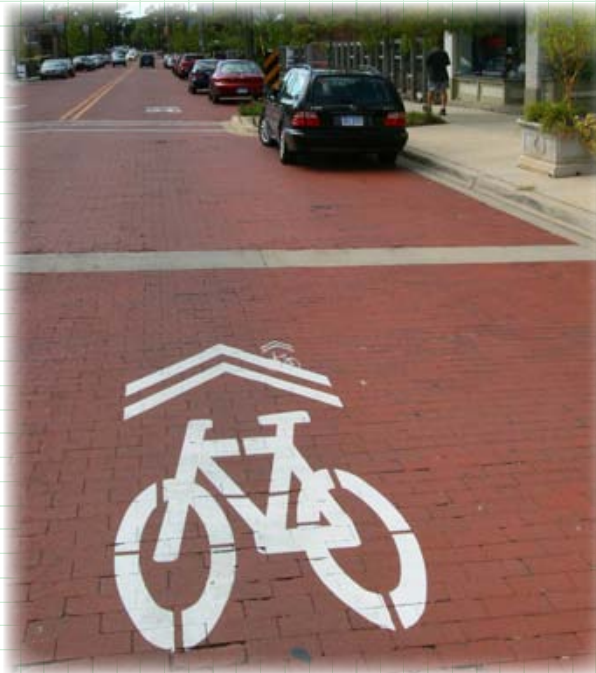
Sharrow Pavement Markings
