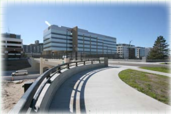
Coit Bridge Reconstruction
