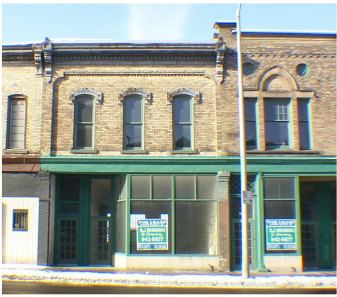
135 South Division, before
