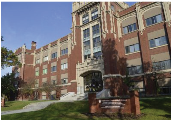
Innovation Central is the oldest continuously used high school in Michigan
