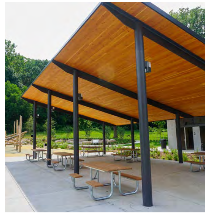
New picnic shelter with accessible picnic tables.
