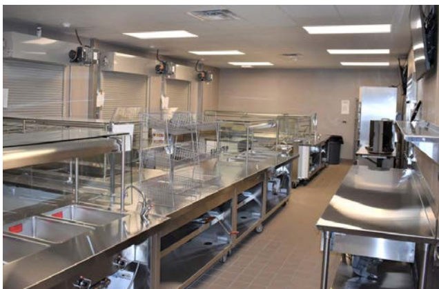
A new kitchen is ready to serve students at OHHS.
