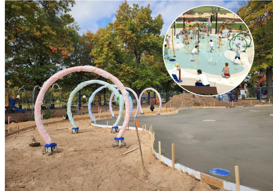
Construction progress at Garfield Park splash pad
