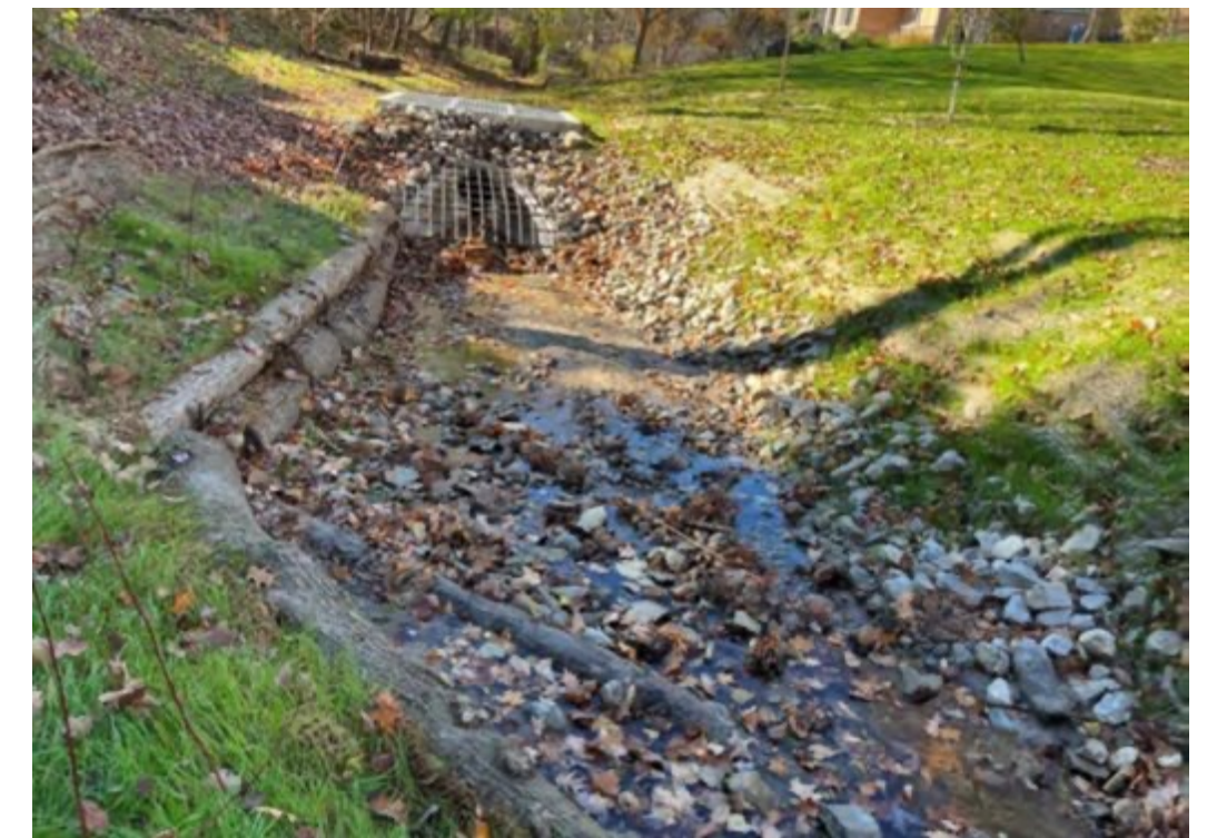
Burton Breton Drain Restoration
