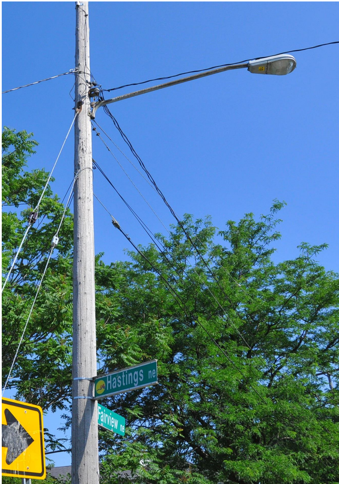
P1 Wood Pole with Cobra Head Luminaire
